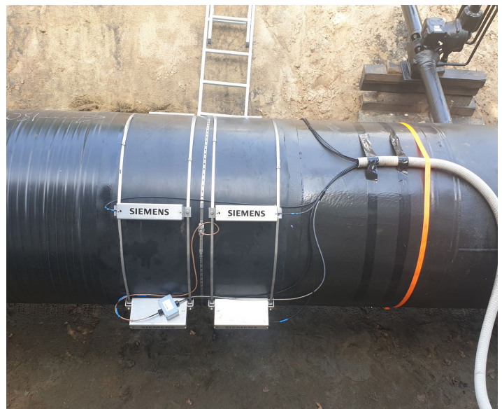
Figure 5: Clamp-on flow meter SITRANS FS230 system components and natural gas flow measurement application with "Soundcoat" to enable operations at low amplitude signals found in gas measurement
